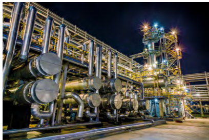
Morning Star Packing, 24 Single Stage Steam Turbines California, USA
