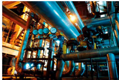
KNPC New Refinery Single Stage, Mechanical Drive steam turbines Kuwait
